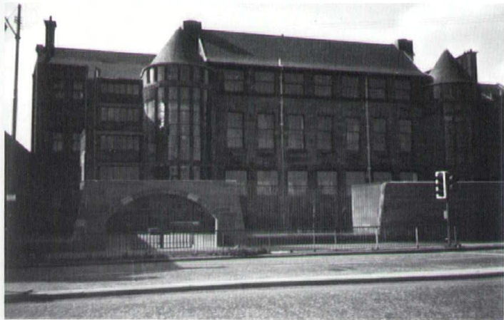
Scotland Street School, Glasgow.
