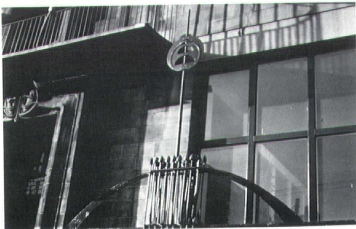
Detail of iron finial, Glasgow School of Art.
