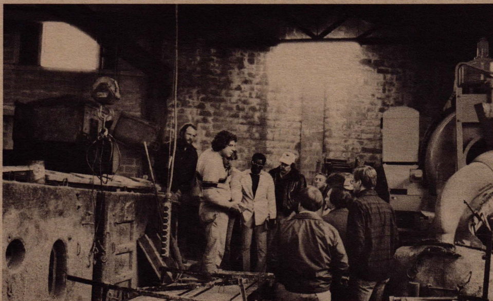
RESTORE workshop session held at Loudino Stone Co. Bill Loudino, a RESTORE student, is showing how a stone ballustrade is produced in the shop.
