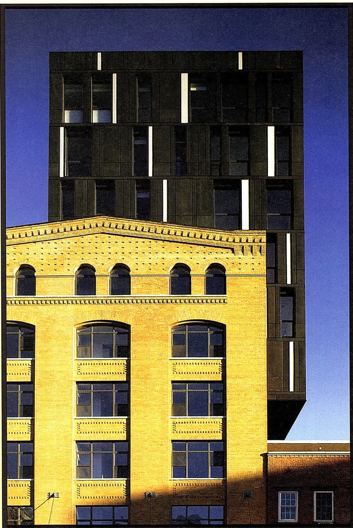
Four new stories of apartments fit neatly atop the renovated six-story warehouse building
