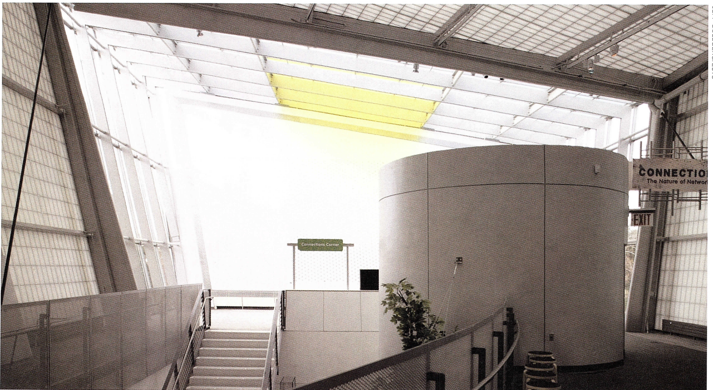
Translucent insulating fiberglass admits daylight in and cuts lighting costs at the Hall of Science
