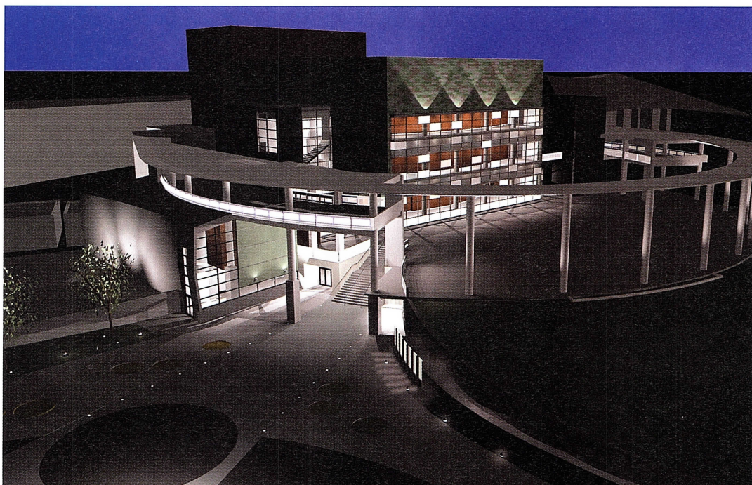
Above: TeamHaas Architects: The new Long Center for the Performing Arts will incorporate the 290-foot steel perimeter support ring of the 1958 Palmer Auditorium Below: Palmer Auditorium today
