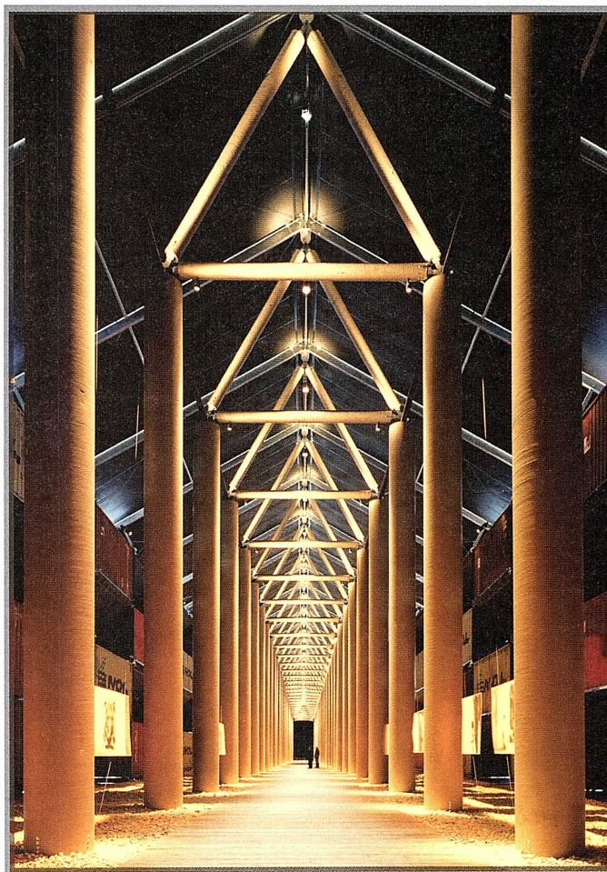
Left: The Nomadic Museum stretched 672 feet along Pier 54 Above: Paper tubing made up much of the roof trusses and columns Below: Axonometric
