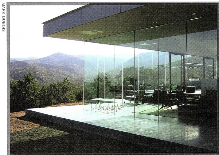
A structural glass wall is the only support for the cantilevered roof over the living room
