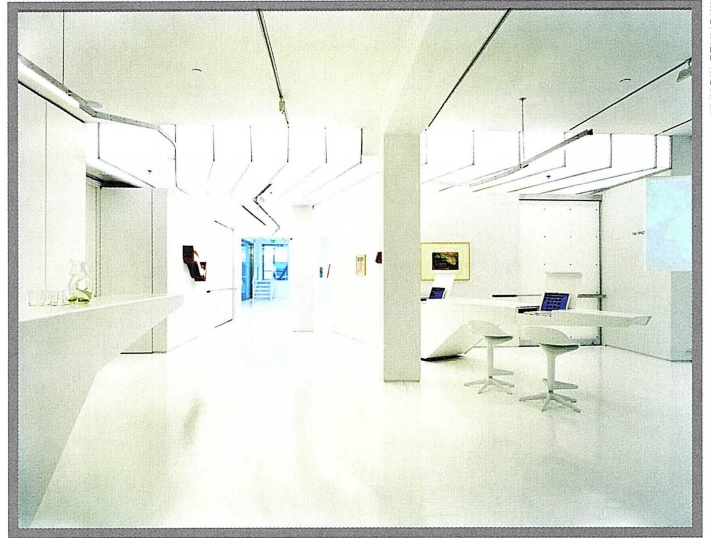
The translucent paneled ceiling houses HVAC and sprinkler systems
