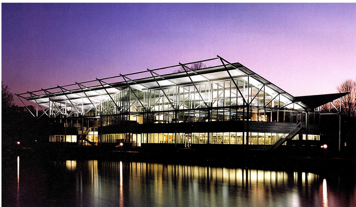
Left: Hellmuth, Obata + Kassabaum: LEED Gold-rated Winrock International HQ, Little Rock, AR: a multifunctional roof controls shade, captures rainwater, and directs enough daylight into the upper floors to make artificial lighting unnecessary year-round Below: weisz + yoes architecture: Jonathan Rose Companies: an office expansion maintained the aesthetics and green material specifications of the initial design by Paul Segal Associates; the design team included Jonathan F.R. Rose and Lisa Tilney of Jonathan Rose Companies
