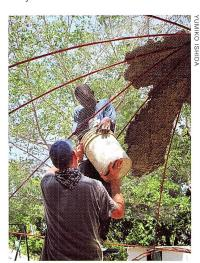
Nura domes, created by Love for Haiti. can be covered with tarp or other materials; this photo shows an experiment in covering one with plaster
