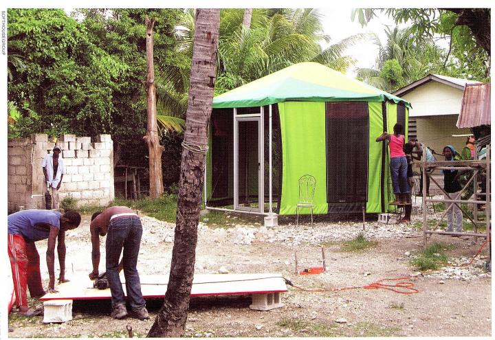
Designed by the SOFTHOUSEgroup, the HaitiSOFTHOUSE consists of hexagonal steel-frame modules that can be combined to serve many different programs over time; ecofriendly elements include rainwater collection and waterproof fabric panels that, when no longer needed, can be reused as material for raincoats or purses
