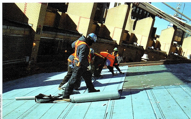
(above) Installation of a vapor barrier in preparation for a new energy-efficient roofing system at Madison Square Garden. New and replacement roofing systems must comply with the New York State Energy Code for items such as R-value (the assembly's thermal resistance or ability to insulate).
