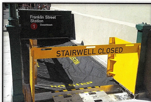
Stairwell Flex Gate® installed & deployed on a NYC subway street level entrance
