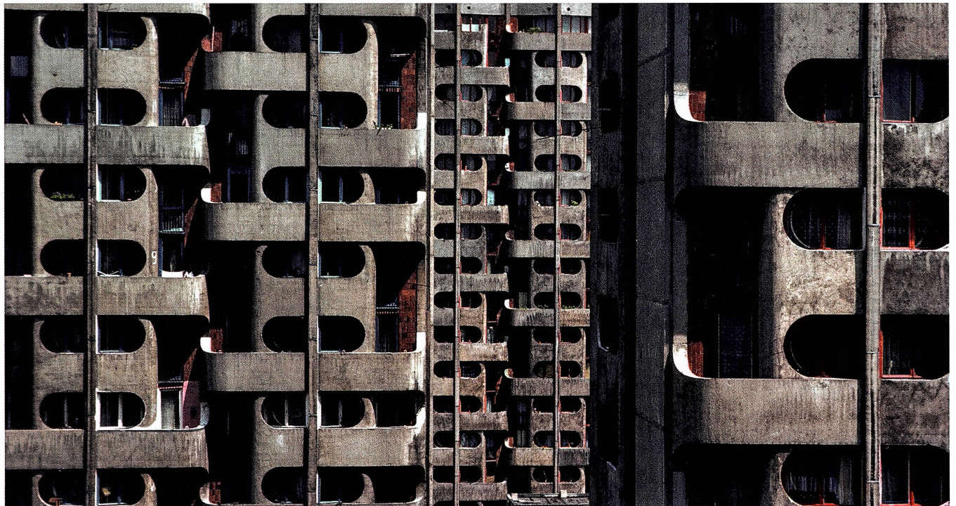
Grabowska-Hawrylak’s iconic residential buildings, pictured here in 1982, were built between 1963 and 1969 in Wrocław’s Grunwaldzki Square.
