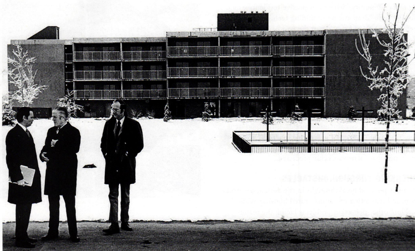
Secretary Romney reviewing completed Operation Breakthrough housing in Kalamazoo, Michigan, one of nine sites ultimately awarded with building contracts
