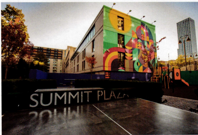
An Operation Breakthrough development that was rehabilitated in 2018, Summit Plaza is Jersey City's largest privately held Section 8 housing complex, comprising a 483-unit property for senior and vulnerable residents.
