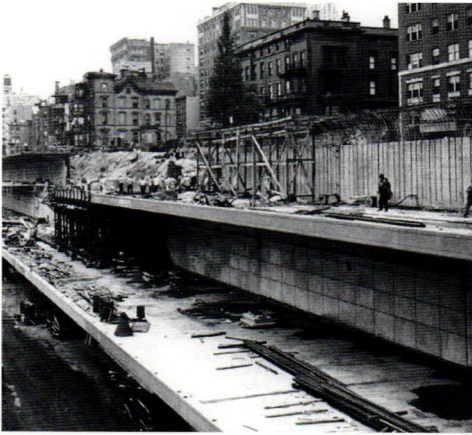
Above: Construction of the BQE's triple cantilever in the 1950s (left) and a photograph of the expressway after its opening in 1954. Above, far right: A model photograph from Linear City, Brooklyn, New York: Feasibility Study and Planning , by McMillan Griffis Mileto, 1967. The model depicts plans for a five-and-a-half-mile linear city, composed of a spine of schools and housing, that would sit atop a pedestrian platform built above a new Cross-Brooklyn Expressway.
