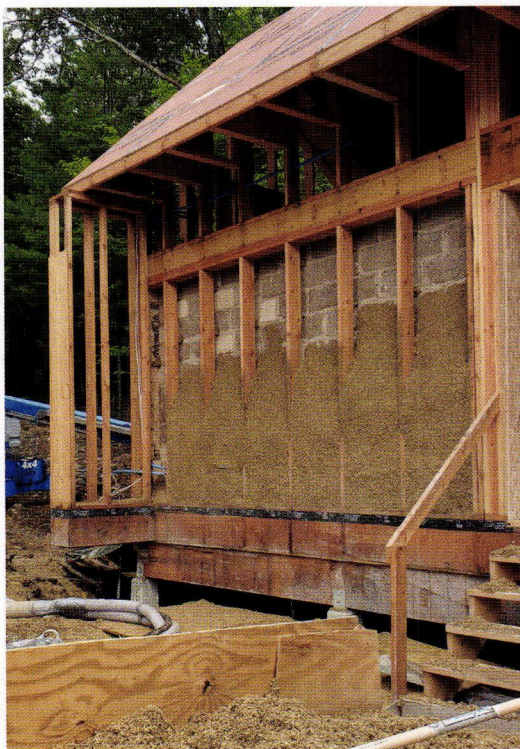
Prefabricated and pre-dried hemplime blocks form an interior layer of continuous insulation. An additional layer of hemplime was sprayed on the blocks and in between the structural frame.
