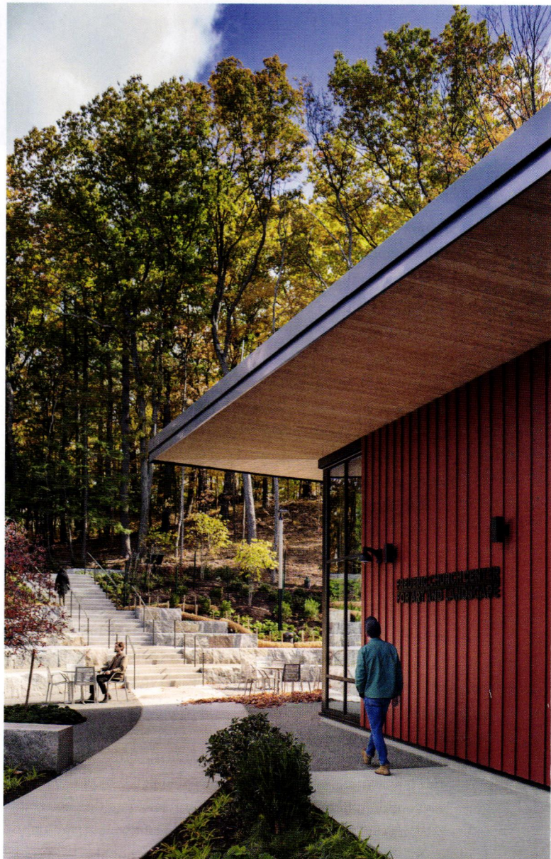
The mass timber center—the first public building of its kind in New York State—has dark red vertical wood siding and generous eaves.
