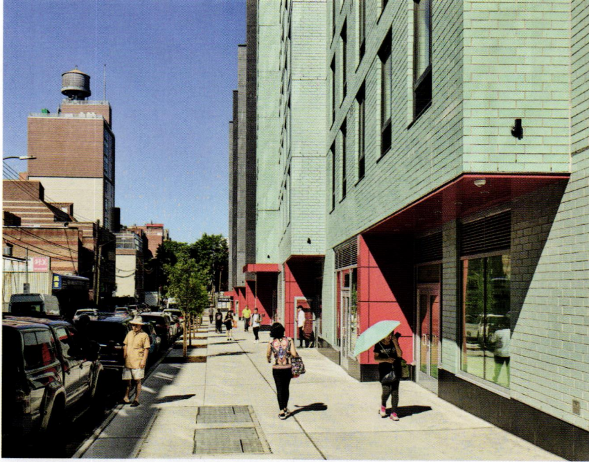
Facing: KPF's New York Office. A careful sense of material craft is part of the firm's design DNA. Above: OneFlushing, designed by Bernheimer Architecture, is a 230-unit intergenerational and all-affordable housing development in Queens, NY. The project includes a 6,000-square-foot community center, providing both adult day care and social-service needs for the neighborhood, and 29,000 square feet of mixed retail space.
