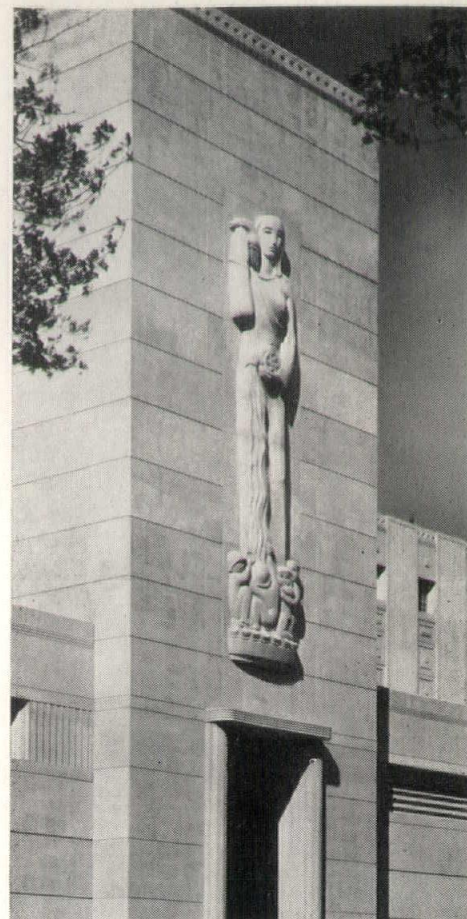
Lansing, Mich., Waterworks. The 32-ft. sculptured figure was formed against a plaster waste mold. Designed by Board of Water Supply and Electric Light Commissioners, Claude Erickson, engineer; Black & Black, consulting architects; Alvord, Burdick & Howson, Chicago, consulting engineers.
