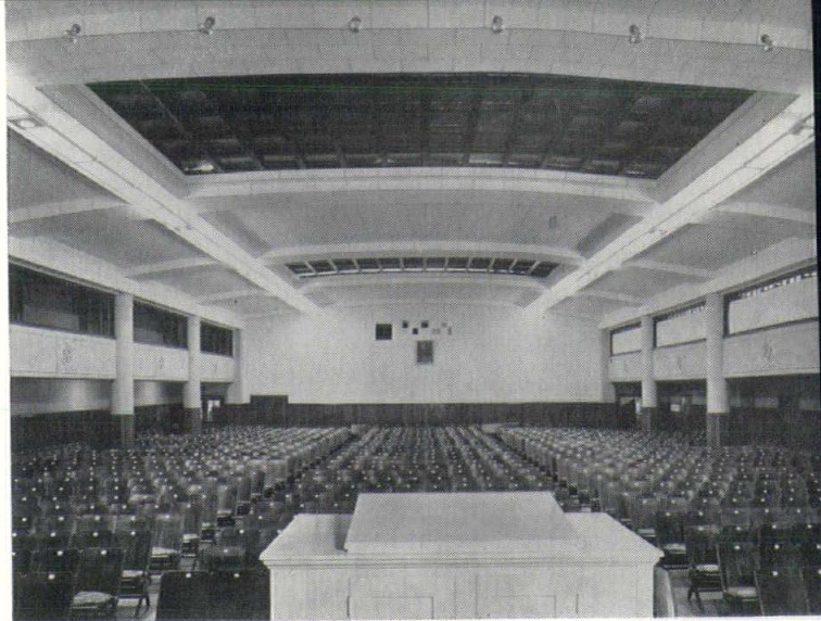
Ceiling and rear wall treatment with perforated fibre acoustical tile, The Temple on the Heights auditorium, B'Nai Jeshurun Congregation, Cleveland Heights, Ohio.
