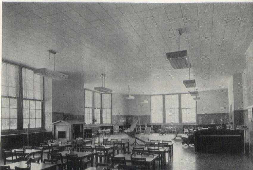
Perforated fibre acoustical tile ceiling in Kindergarten, Ladyfield School, Toledo.
