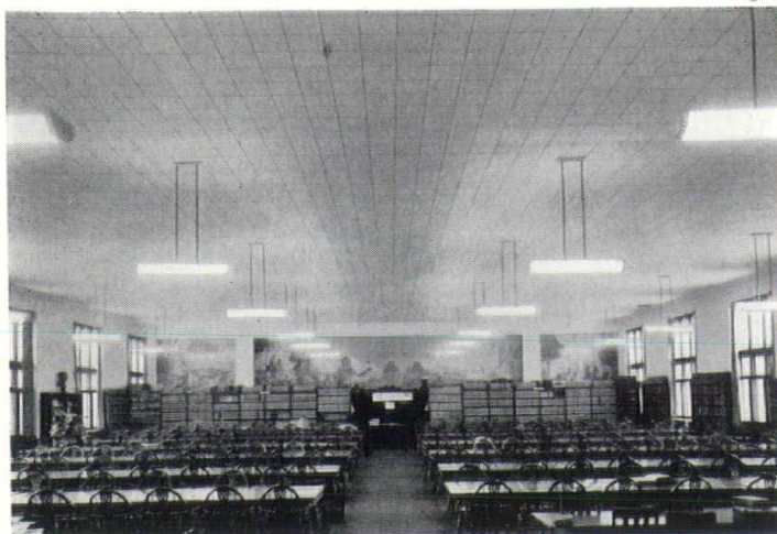
University of Toledo Library, showing ceiling of paintable Acousti-Celotex cane fiber tile, erected with adhesive cement against plaster.
