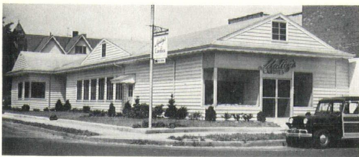
"FIRST IN AMERICA": An example of a completely engineered retail building with all aluminum exterior, insulation and interior trim. 4,000 sq. ft. of air-conditioned comfort for the public and manufacturing areas built at a cost of approximately $15,000 less than with conventional materials. (All aluminum supplied by 'lumiland Distributing Co. Rocky River, Ohio)
