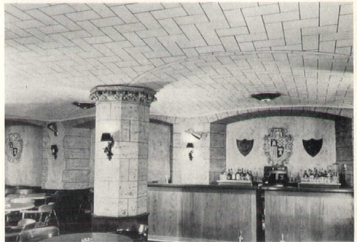
Ceiling of Acousti-Celotex perforated fibre-tile cemented to plaster in the English Grill, George Washington Hotel, Washington, Pennsylvania.
