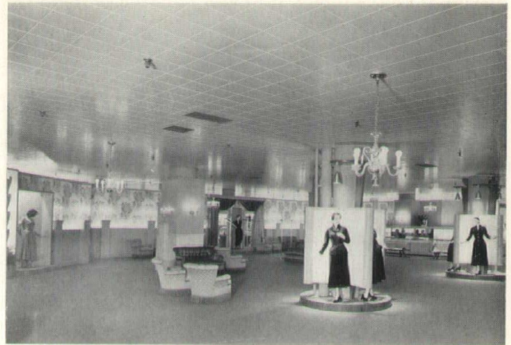
Lindner-Davis Company, Cleveland, third floor. Ceiling of Acoustel Perforated Metal Tile with air-flow channels, approximately 33,000 square feet. Architects — Ward & Conrad.
