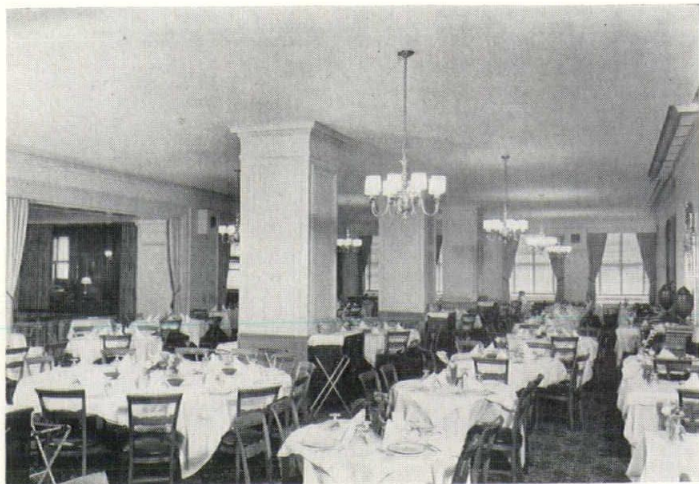
New main dining room ceiling, Cleveland Athletic Club, treated with square-edged units of Celotex Fissuretone, levelled with concealed splines. Architect; Dalton-Dalton Associates.
