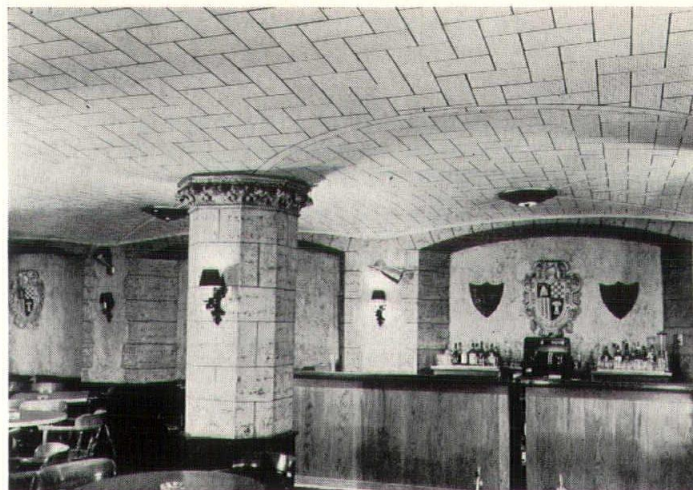
Ceiling of Acousti-Celotex perforated fibre-tile cemented to plaster in the English Grill, George Washington Hotel, Washington, Pennsylvania.
