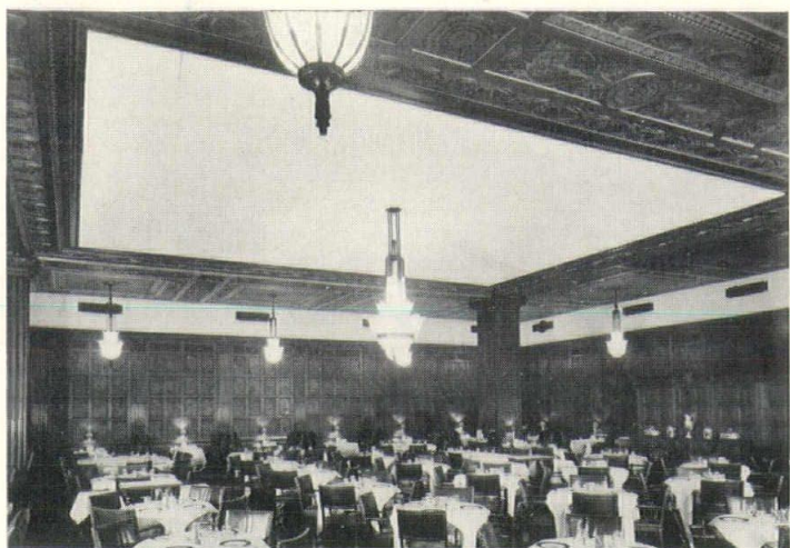
Fred Harvey's Oak Room, Cleveland Union Terminal. Acousti-Celotex applied on ceiling and upper side walls, later stencilled to reproduce former decorations.
