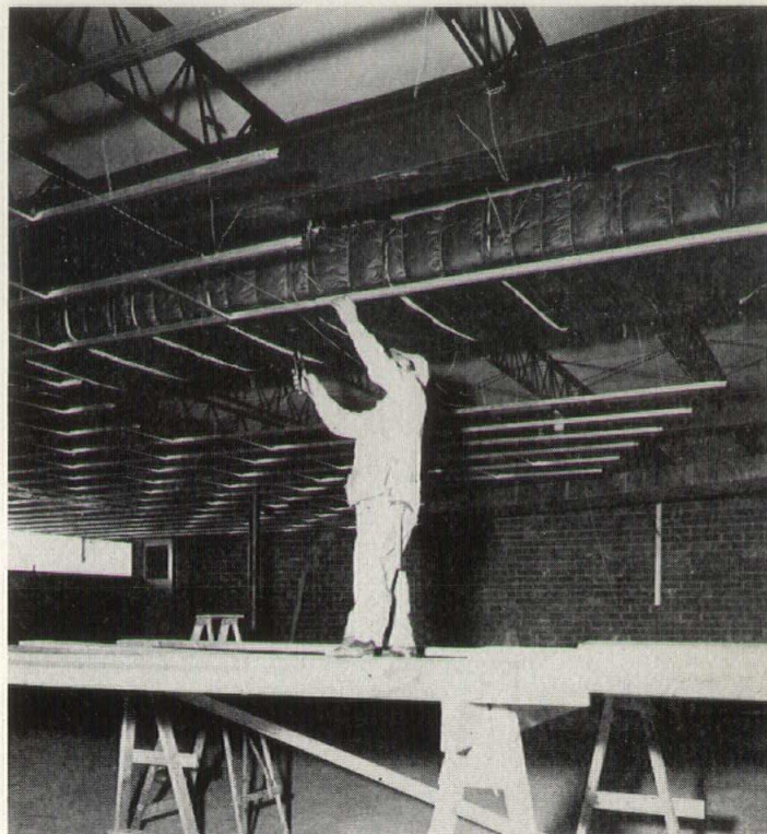
After attaching hanger wires to the structural members, the lightweight grid system is rapidly installed to receive Fibreglas Ceiling Board. The extensions are fabricated on the ground and easily joined with a pair of pliers.
