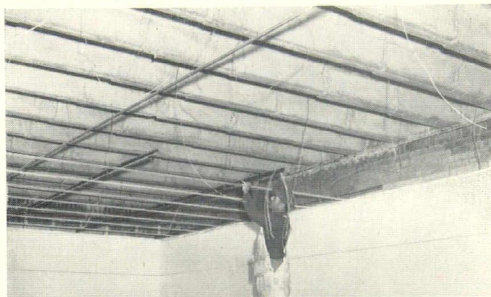
Gilles-Sweet School addition classroom. Workman ties I-Runner to 1 1/2" carrying channel. Note rod hangers used to tie carrying channel at ceiling level. Perforations along the aluminum I-Runner web enables workman to tie runner-to-channel anywhere along runner's length.
