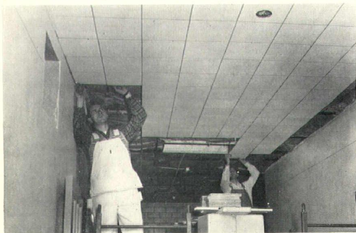
Workmen attach tile to I-Runner in upstairs corridor. Direct-to-metal acoustical tile application is done by placing kerfed edges of tile over lower I-Runner flanges. Tile are interlocked by means of lateral-supporting Reinforcement T-Splines. Use of all-aluminum suspension system with glass-fibre tile provides non-combustible ceiling installation.
