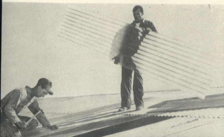
Installing Corrugulux skylights in existing building
