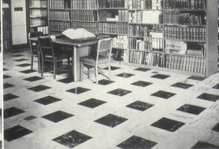
The floor in this library is of Terraflex, made of vinyl resins and asbestos fiber, it is a resilient flooring that is quiet underfoot.
