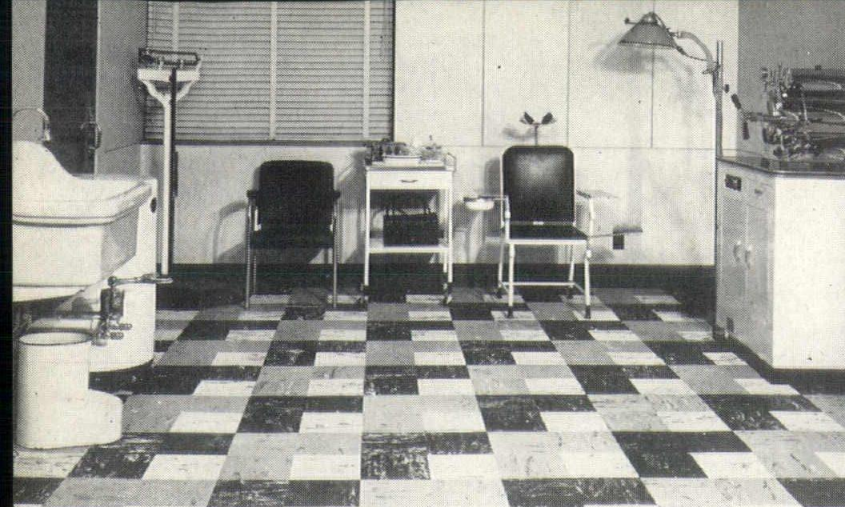
The floor in this medical room is of Terraflex, the new plastic-asbestos floor tile. It is not harmed by mild acid solutions and disinfectants used in hospitals, etc. It is available in twelve attractive colors.
