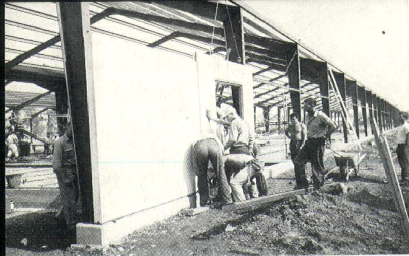
Marietta panels were of two basic sizes — 8' x 10' x 5" and 8' x 8' x 5", plus special sizes. Window frames were cast into panels.
