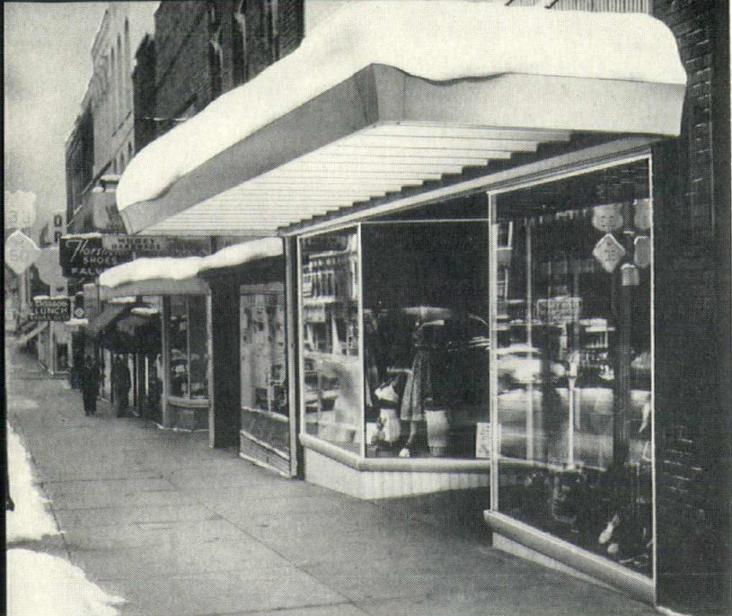
Building owners need not fear the effects of accumulated snow as shown on the above marquee. Laboratory tests proved it will stand up under a load of 60 pounds per square foot, which will meet maximum building code requirements.
