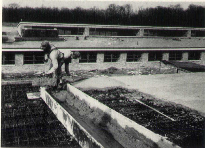
The lightweight perlite concrete is light enough to be easily shoveled from the end of the trough to the surrounding area. It can be wood screeded to a smooth, even surface without the additional labor of steel trowelling.
