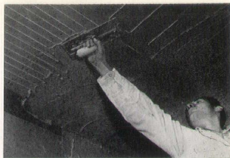
Sunwarm cables are completely concealed under ceiling plaster, which should be allowed to dry before current is turned on.
