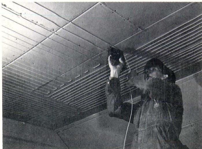
Sunwarm Radiant Heating Ceiling cables are stapled to ceiling before plastering. Experienced electrician can complete average room in one hour's time.
