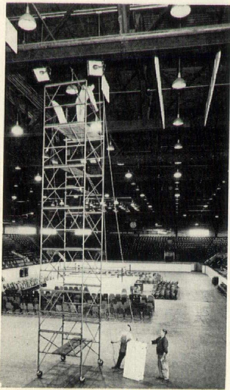
Installation of more than 3,000 Fiberglas Noise-Stop Acoustical Baffles in the Toledo Sports Arena was completed by the arena's own maintenance crew. Workmen are shown as they raise the "packages" of baffles to the top of a scaffold, where they were hooked over wires strung under the ceiling. Each baffle weighs only six pounds.
