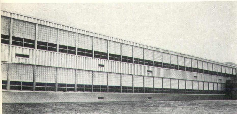
**Close-up view of Mahon "Fluted" Insulated Metal Wall showing Coping Detail of parapet wall.**
