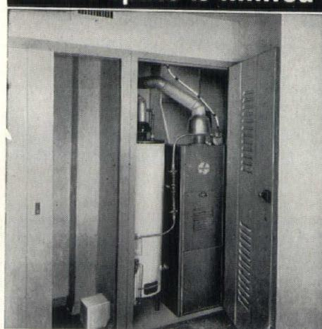
One of a large family of Niagara gas, oil and coal furnaces, the gas-fired Model 10-50, shown here, occupies only 16"x23" floor space. Thousands are doing yeoman service installed in "clothes closet" space together with a water heater.
