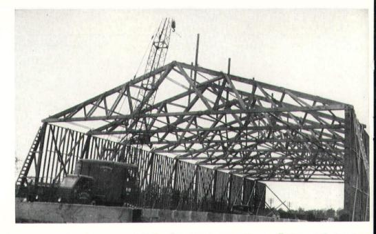
Typical timber-connector roof trusses and columns for low-cost warehouse construction near Schenectady, N. Y. Note provisions for wind loads by use of A-frame columns on one side of building. This frees interior for crane operations. Entire roof structure and wall framing furnished and erected by Cartwright & Morrison, Inc.
