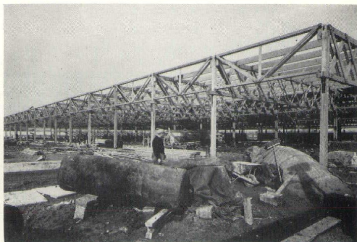
Photograph of timber-connector roof structure by Cartwright and Morrison, Inc., Holcomb, N. Y., for warehouse at Fairlawn, New Jersey. Building is 370 ft. wide by 405 ft. long, truss spans 61'-6"; columns on 22 ft. centers. Purlins are 4 x 16 timbers on 8 ft. centers, with 2 inch d. & m. decking directly over.
