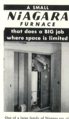
One of a large family of Niagara gas, oil and coal furnaces, the gas-fired Model 10-50, shown here, occupies only 16"x23" floor space. Thousands are doing yeoman service installed in "clothes closet" space together with a water heater.
