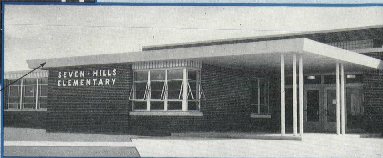
This entrance canopy provides a distinctive highlight for the Seven Hills Elementary School, Seven Hills, Ohio, adding design interest to the building. Canopy fascia and soffit as well as the gravel stops are of Davidson Architectural Porcelain. Architects: Fulton, Krinsky & DeLaMotte, Cleveland.
