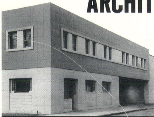
American Sales Company office, Columbus, Ohio, shows use of Davidson Architectural Porcelain for building facade and ribbon-type window treatment. Architect: Leon Seligson, Columbus, Ohio.
