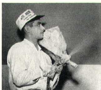
Hushkote ceilings and sand finished sidewalls all finished with Plaster-Tex machine.
