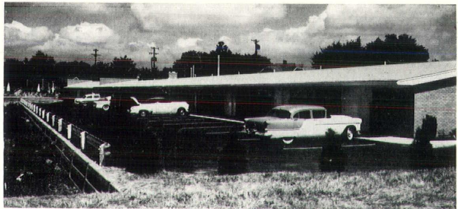
Partial view of Terrace Motel, Dayton, Ohio, showing the installed Armco Bin-Type Retaining Wall at the left. Armco FLEX-BEAM Guard-rail is mounted on top.
