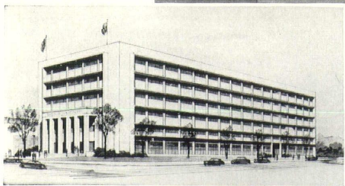
National Cash Register Engineering and Research Building has Flexicore electrified floors. Architects, Lorenz & Williams. Consulting Mechanical Engineers, Schweiger, Heapy & Associates.
