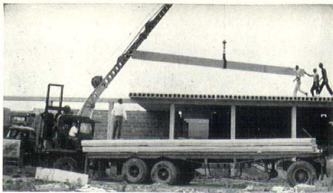
Firesafe concrete roof is erected in a few days. Flexicore roof slabs are precast in factory, keep costs low, save on-the-job labor.
