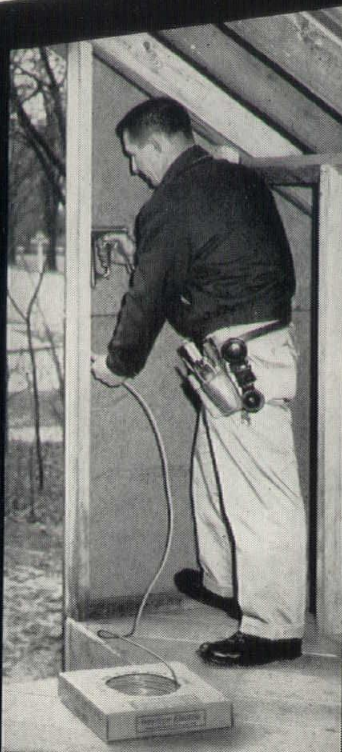
Pre-wiring easily done when homes are being built.
