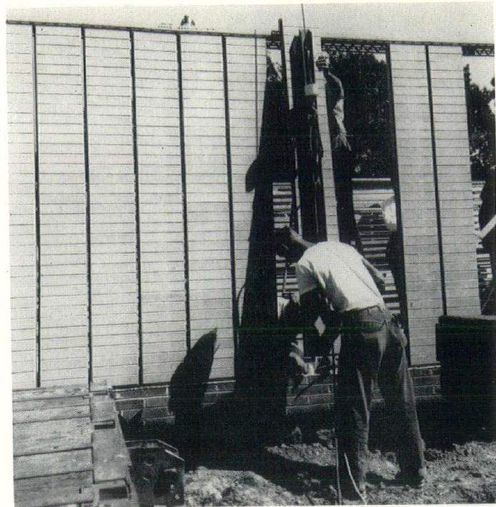
A new prefabricated brick panel, two and one-half inches thick, called the "SCR building panel"*, has been successfully used in the construction of a full-size ranch style home here.
