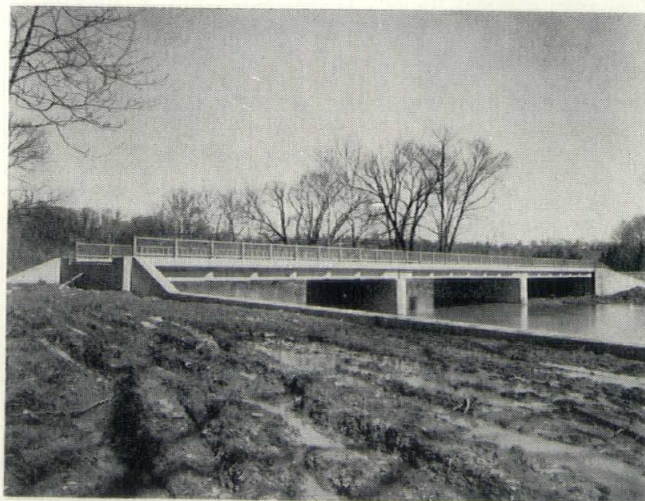
Rocky River Reservation Bridge utilizes 54 prestressed concrete beams.
