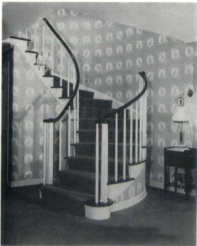
Shipped entirely assembled was this exquisite staircase for the home of Miss Darthea Rowland, Franklin, Pa. Millwork was built up at Hyde-Murphy plant in Ridgway, Pa. Note rosette where rail butts into wall and 180-degree turn of left rail. Spacious effect is enhanced by use of full-length mirror facing base of staircase.
