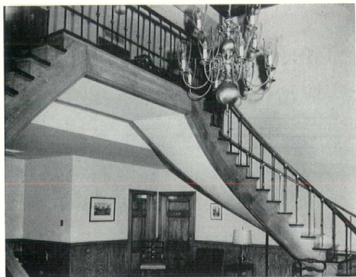
Broad white fascia, intricately lathed balusters, use of the quarter turn and breakover provide opulent beauty for Dr. Magee's home. Hyde-Murphy designed staircase and mezzanine handrail to blend harmoniously into the general architectural scheme.
