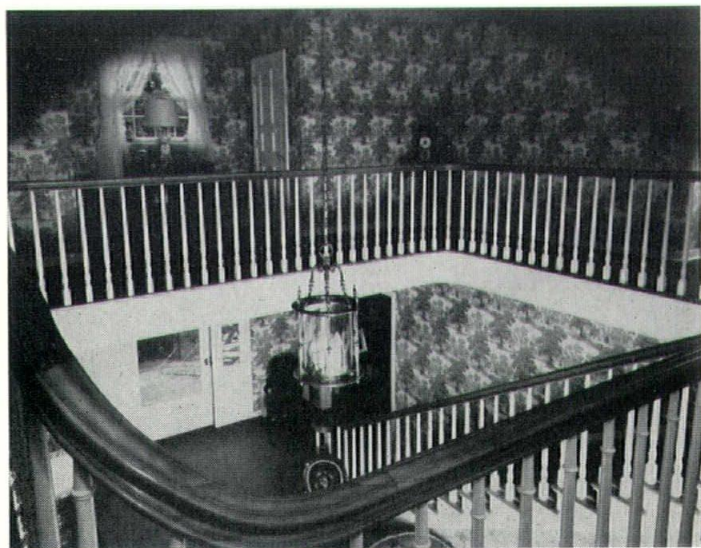
Gently curving twin stairways in the lobby of the Asphalt Institute Laboratory, University of Maryland, feature handrails of straight-grain walnut and risers, stringers, and platform skirting of white pine, finished natural. Treads and nosings are marble.
