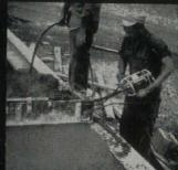
Spud Vibrating Stems and Screed Vibrating Flanges
