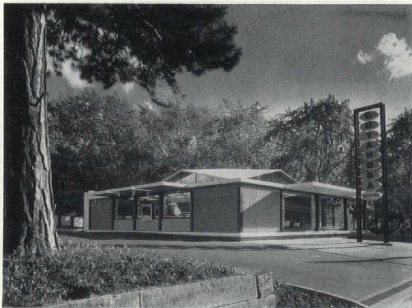
Architects: Dalton-Dalton Associates, Cleveland • for Cuyahoga Savings Association
