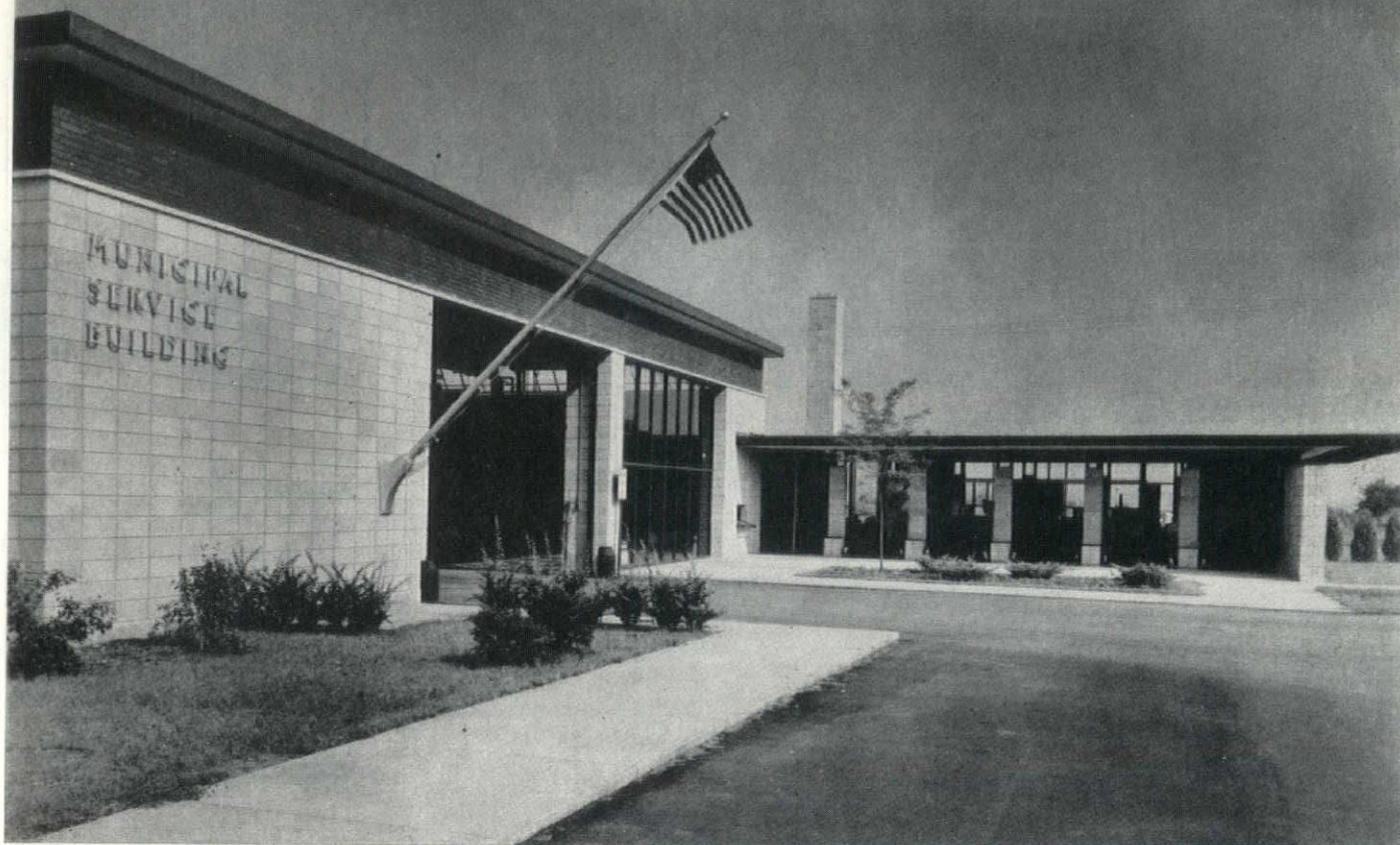
Walls are stacked concrete blocks with burnt brick cornice band. Copper fascia trims Flexicore roof overhang.
