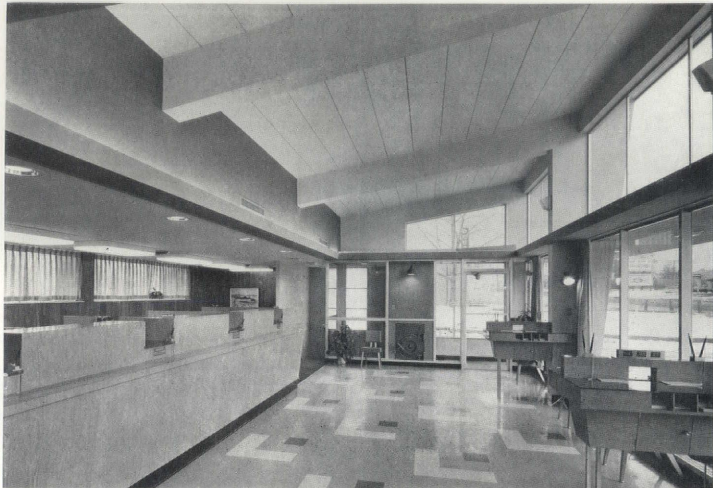
Bank of Akron at Cuyahoga Falls has Flexicore floor and inclined roof, with exposed ceiling.
