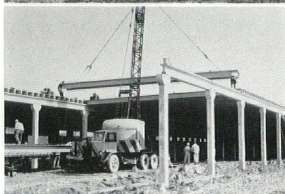
Work crew installs precast roof slabs at rate of 1000 square feet an hour.
