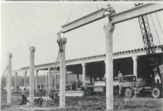
Two men with motor crane quickly install precast roof beam on concrete column.
