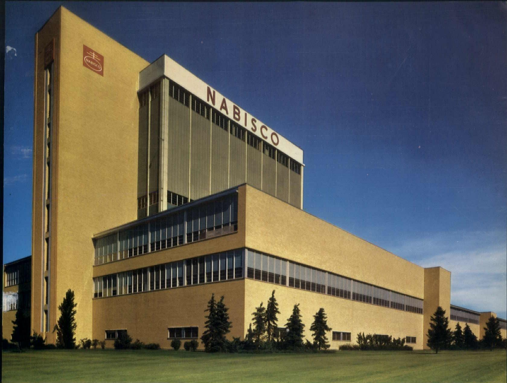
The National Biscuit Company's Fair Lawn, N.J., plant, showing exterior walls of Natco Dri-Speedwall tile.
