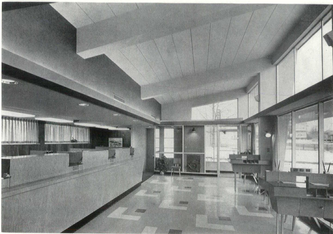
Bank of Akron at Cuyahoga Falls has Flexicore floor and inclined roof, with exposed ceiling.
