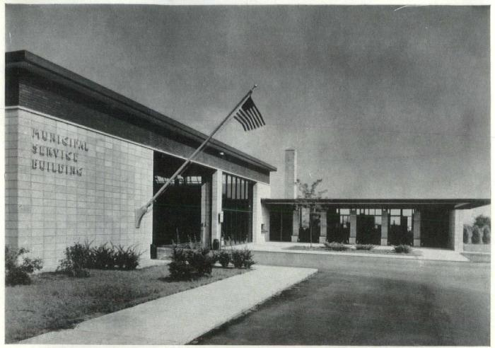
Walls are stacked concrete blocks with burnt brick cornice band. Copper facia trims Flexicore roof overhang.
