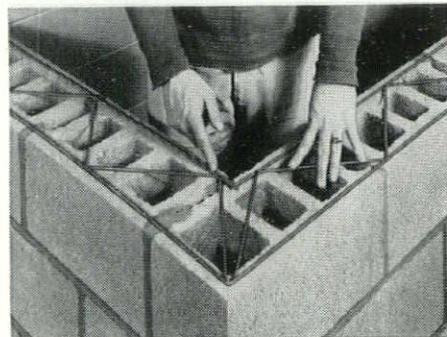
*Two engineered products that meet a need. Dur-o-wal reinforcement, shown above, and Rapid Control Joint, below. This ready-made control structure flexes with the wall. Recommended by construction engineers especially for concrete block.*
