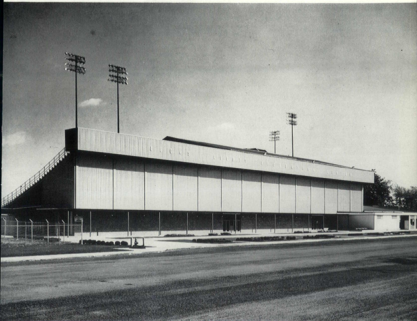
Remodeled Grandstand showing increase in size and galvanized asbestos siding applied over old and new Grandstand. Photo by Walbridge & Bell, Inc.
