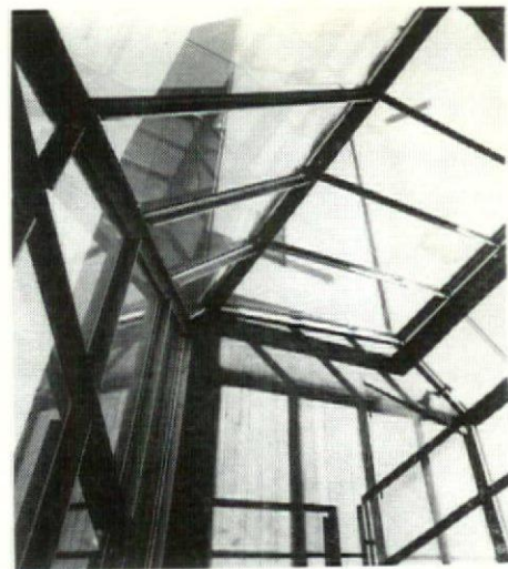
A detailed view showing the aluminum glazing bars in the Engineering Building at Leicester University.
